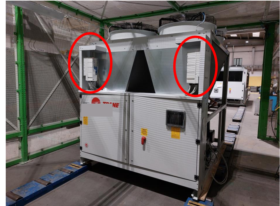
Housing of inverters device for pumps (digit 37)
